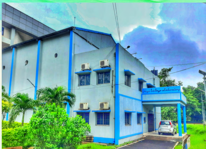
High Voltage Laboratory
